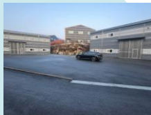
South Korea Manufacturing Factory
