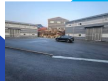
South Korea Manufacturing Factory
